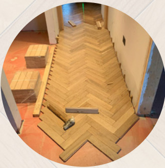
Timber Floor Installation
